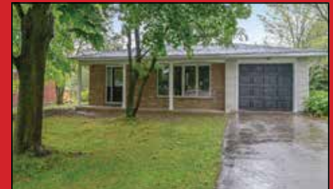
Renovated Erin Backsplit
