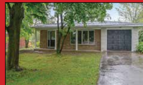
Renovated Erin Backsplit
