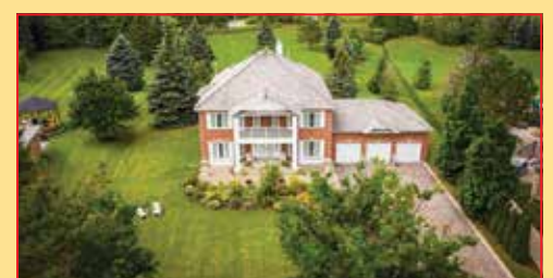
RENOVATED 2 STOREY HOME ON ACRE LOT! $2,850,000 Renovated home on acre lot in prestigious "Preston Lake Community" with access to private lake. Approx. 4800 sq. ft 2 storey home with 2 storey dining room!
