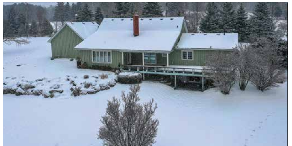
21 ACRES WITH CUSTOM HOME & AMAZING VIEWS This estate bungalow features 3 bedrooms, 3 bathrooms, updated kitchen with marble top island, open concept family/living area & part finished walkout basement. Huge covered deck, paved driveway, 2 car garage plus large workshop. 247515 5th SIDEROAD, MONO $2,499,000
